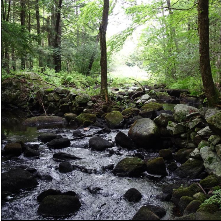
Stone structure crossing Tarbell Brook.
